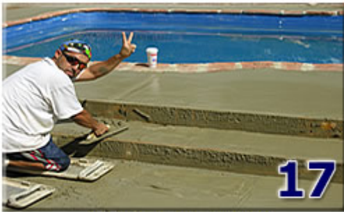
The stairs are poured
