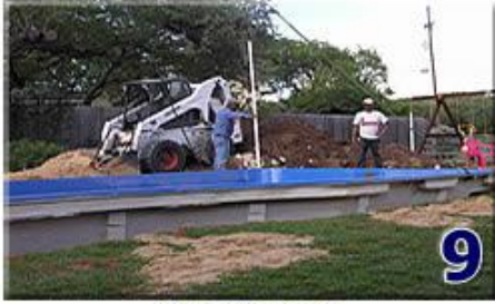
Checking Levels
