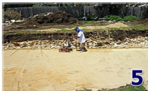
Compacting the bed
