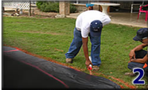
Marking the yard using the template
