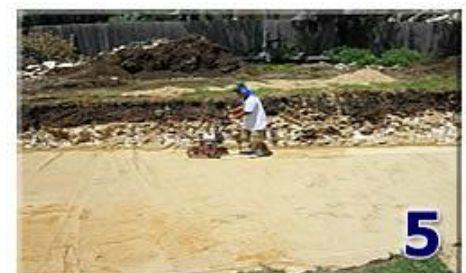
5 Compacting the bed
