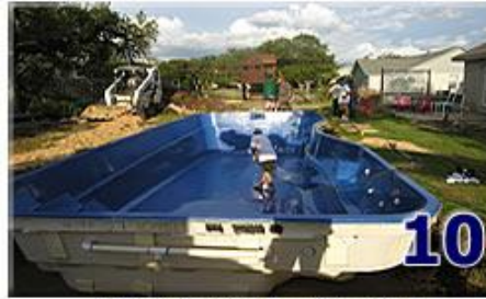
Filling the pool with water
