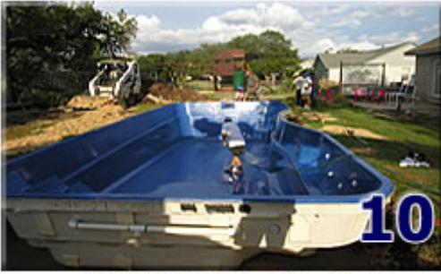
Filling the pool with water
