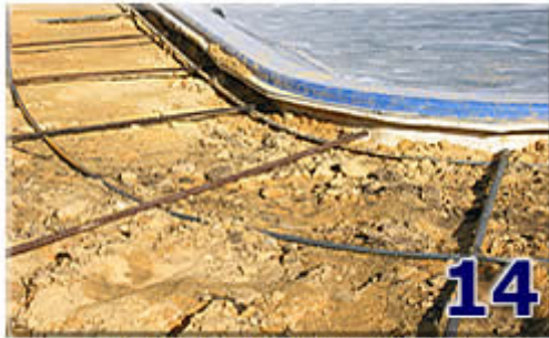
Bonding the Pool and Deck
