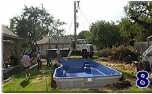
The pool is lowered into the hole
