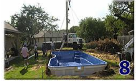
The pool is lowered into the hole
