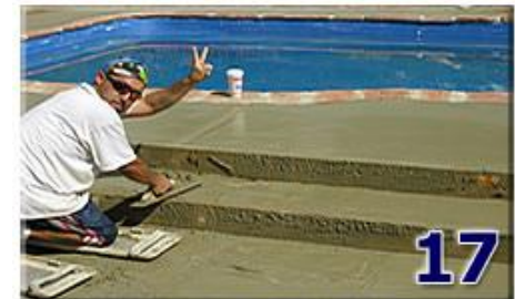
The stairs are poured
