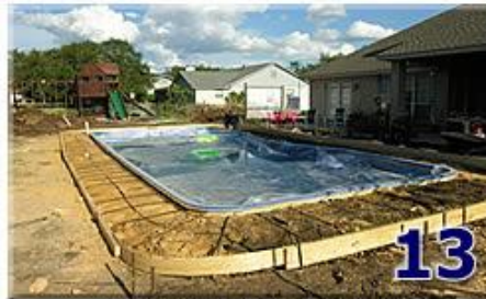
Forming up for the deck
