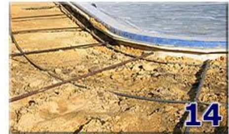
Bonding the Pool and Deck
