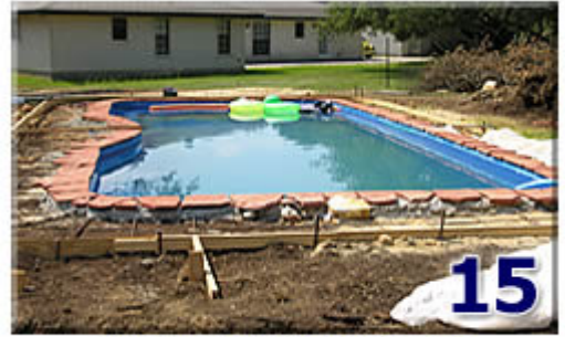
The flagstone coping is laid
