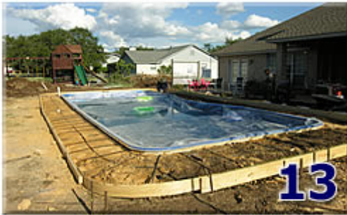
Forming up for the deck
