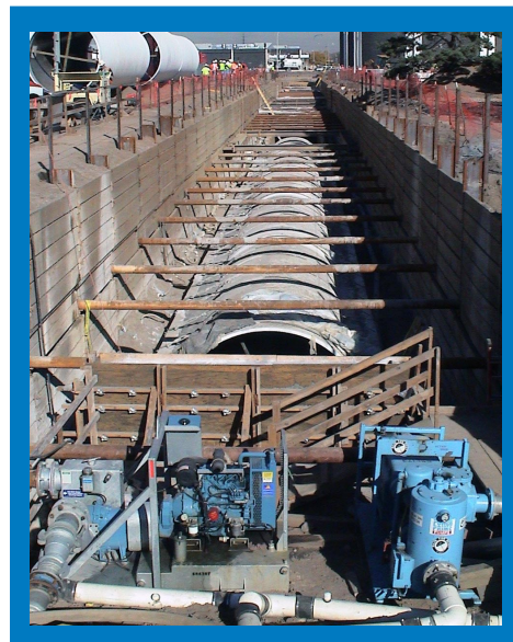
Five hundred feet of composite pipe were installed.
