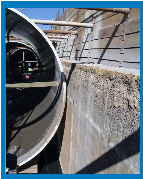
Belco custom-designed the pipe to fit precisely into the "trench" created by removing the damaged portion of the existing concrete culvert.
